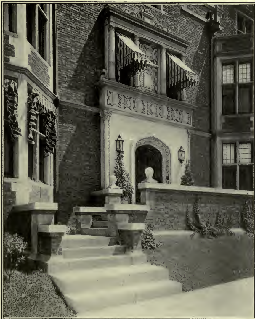
ENTRANCE OF BLACK RESIDENCE.
